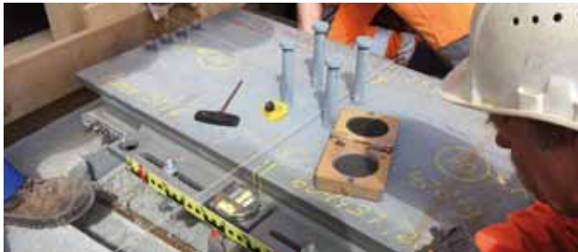
Installation Botlekbrug, Netherlands
