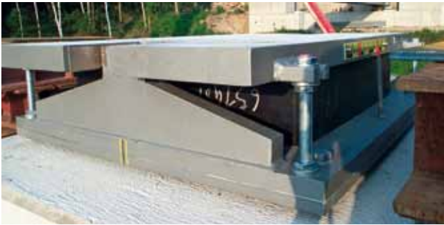
MAURER Elastomeric Bearing
