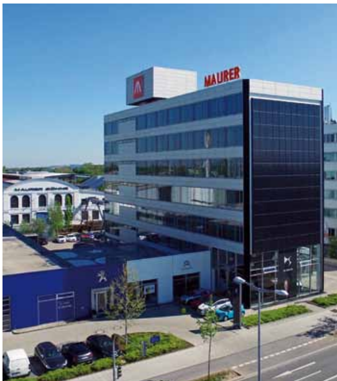
MAURER headquarters, Munich / Germany
