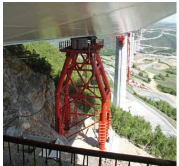
Balancelles Viaduct, Millau / France
