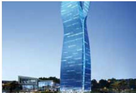
TUNED MASS DAMPERS
