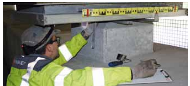
Inspection of bridge bearings
